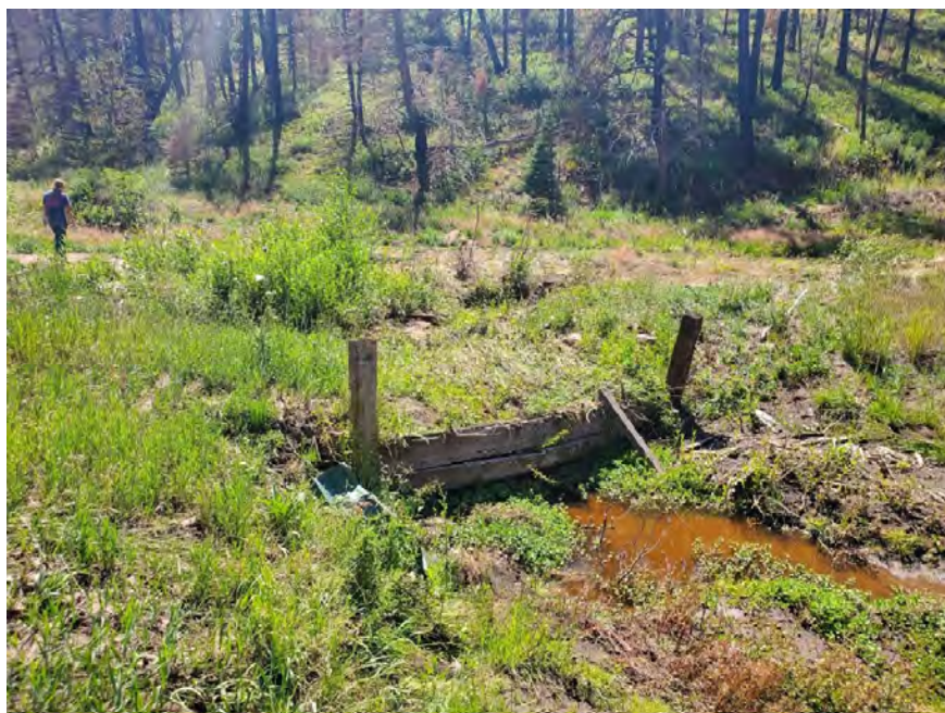
Figure 9: Existing wood check structures along South Middle Creek at Dahmer Fields.
