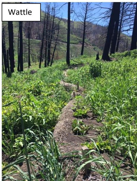
Along Indian Creek, the teams have installed hillslope treatments including 30 wattles, 73 log erosion barriers (LEBs), and 4 crib walls; 8 acres of hillslope on the burn scar have been hand seeded. Wattles were described by Nutter as logs set into the hillside in order to slow the flow of water downhill and “catch sediment to keep it from getting into the waterways.”
